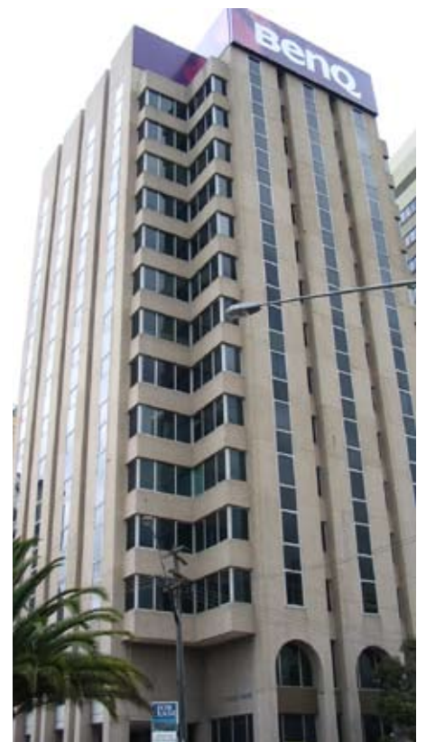
The 1960s Milsons Point building before PTW Architects' innovative adaptation.
